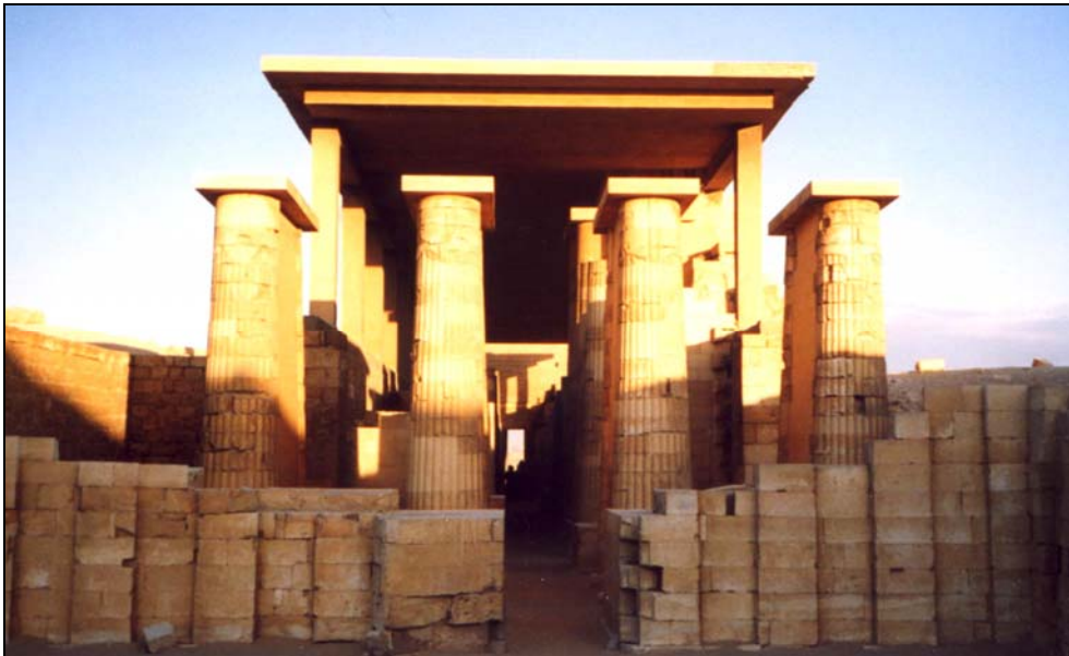
The first pillared hall in the world built out of rock
